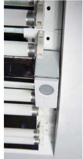
Close-up of Integral Occupancy Sensor in 6 Light Only
