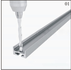
Drill hole for power cord.
